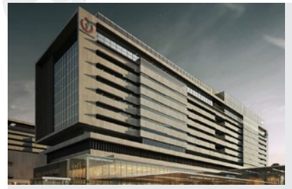
Basaksehir Çam and Sakura City Hospital 4912 Bed Capacity
